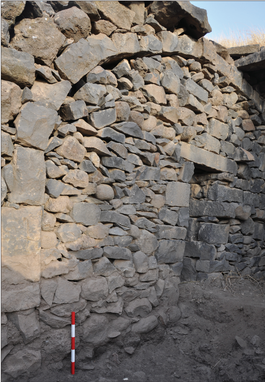
Fig. 6. The stalls along the southern wing of the khān . (Photo by Shai Scharfberg)
