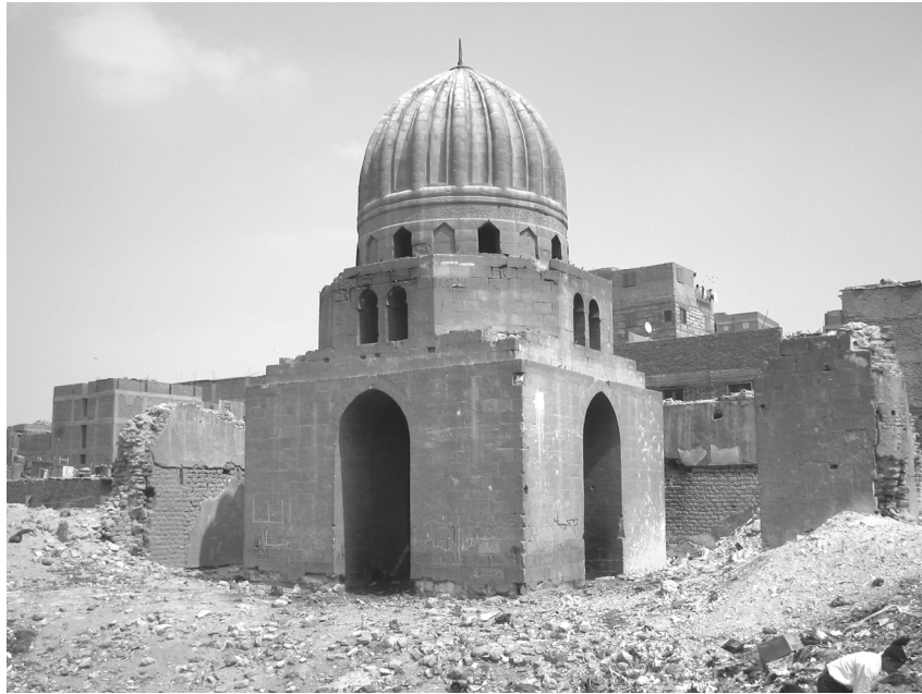
Fig. 7. The dome within the īwān
