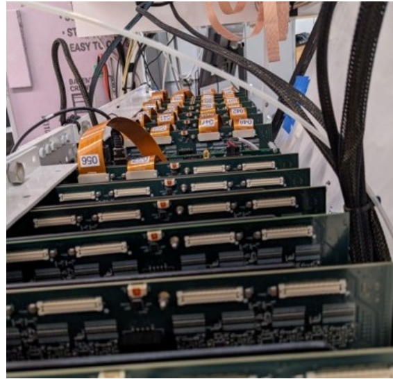
(b) A view of the RICH boards, partially cabled.
