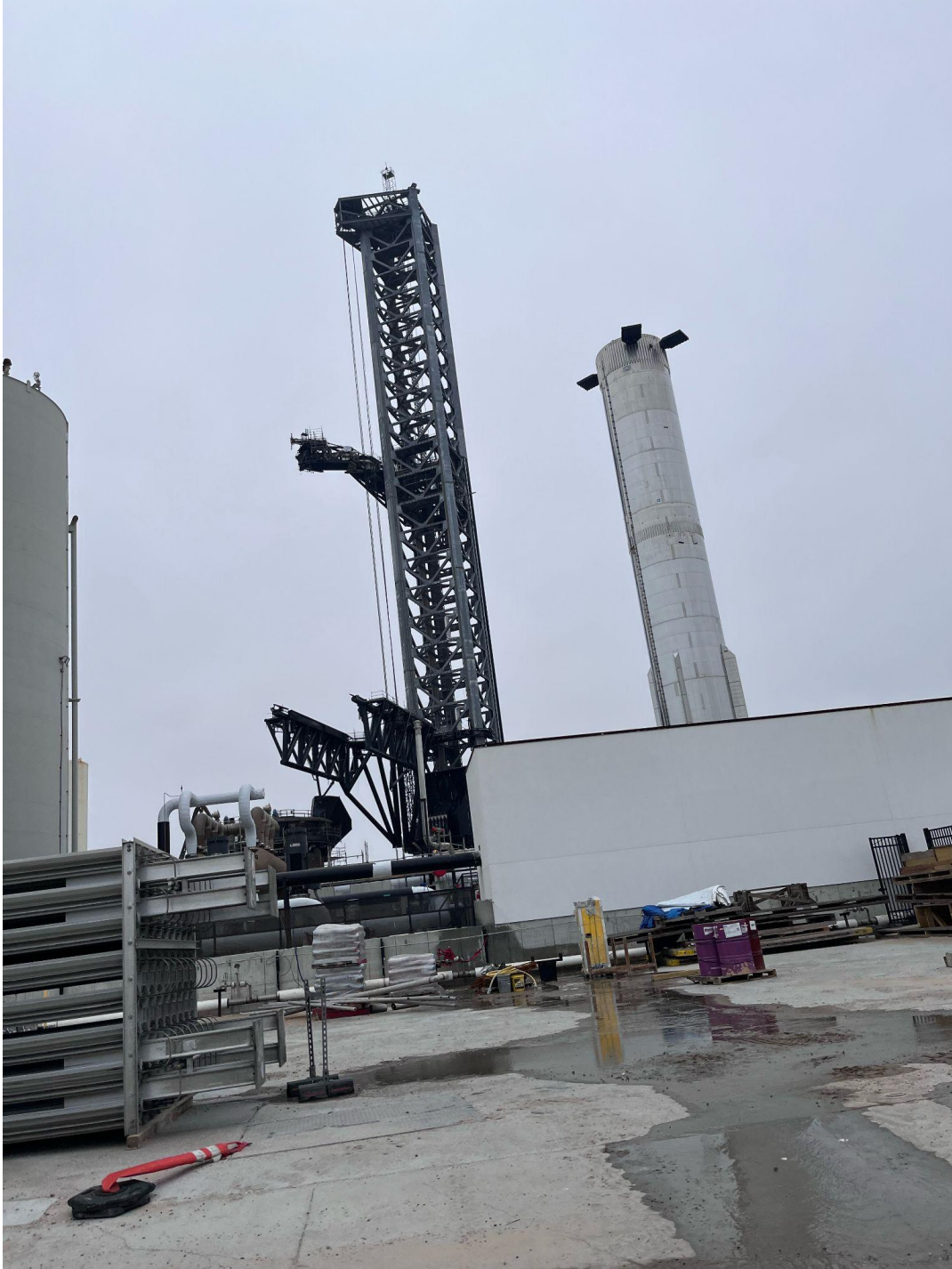
Figure 16: A view from Highway 4 while passing by the Starbase facility.
