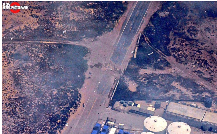
Figure 24: An aerial image of the damage done within the blast range within Starship's launch. (RGV Aerial Photography 2023)
