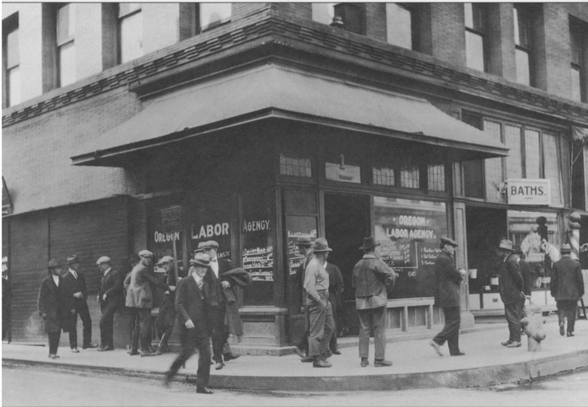
Figure 1. Men standing outside Oregon Labor Agency at the northwest corner of Ankeny and Second in Portland in 1910. Some were reading the information about available jobs such as “dairy man” and “choker setter” on the windows of this employment agency. Such private
