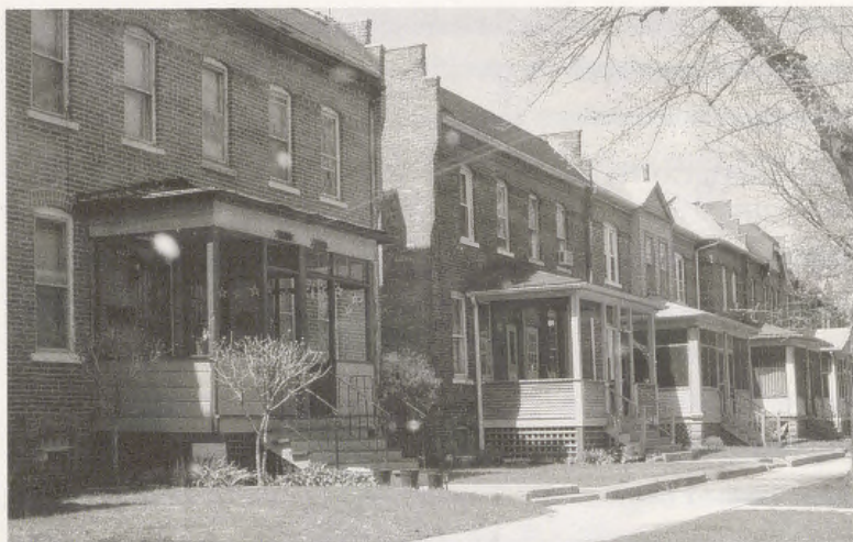
Figure 11. Group of porch additions between 112th and 113th streets.
