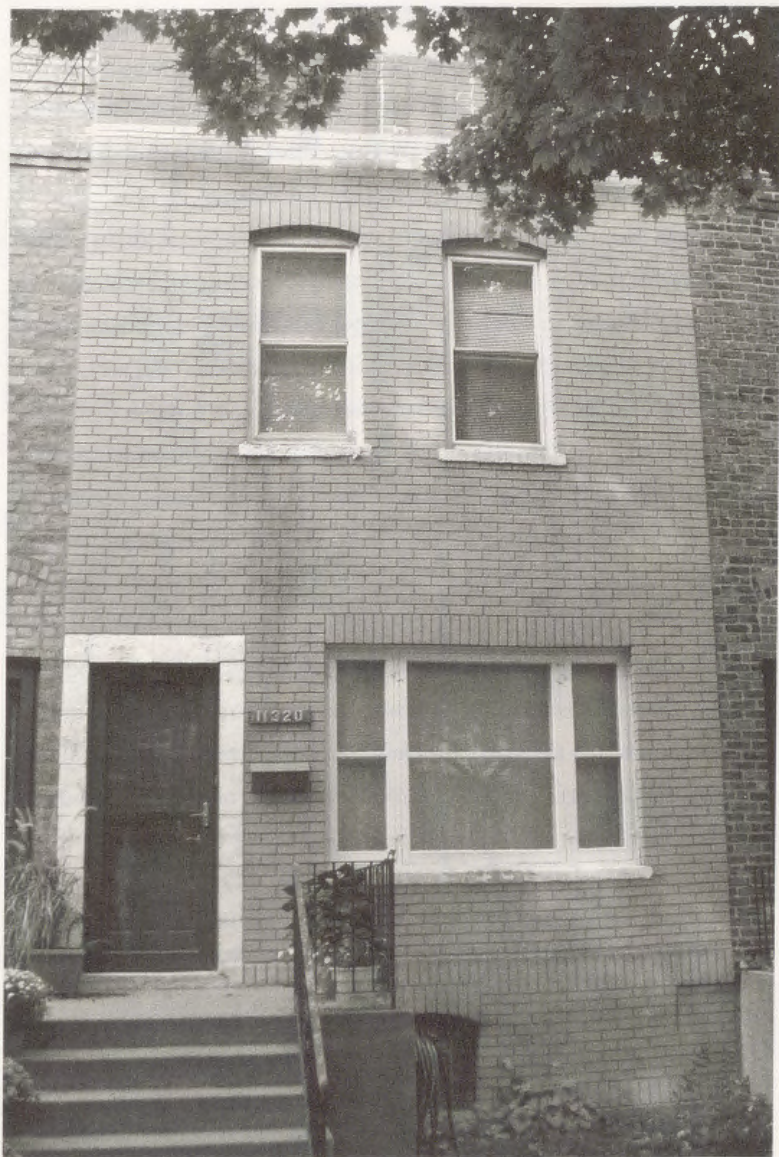
Figure 8. Facade and window modifications on a small row house.
