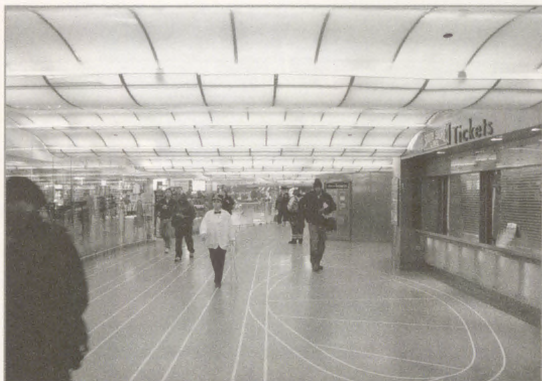
Figure 68. Design of Millennium Station Pedway: note the orienting lines overhead and underfoot, sloping floor, and ceiling light fixtures.
