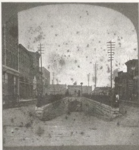
Figure 24. East Entrance of the Washington Street Tunnel.
