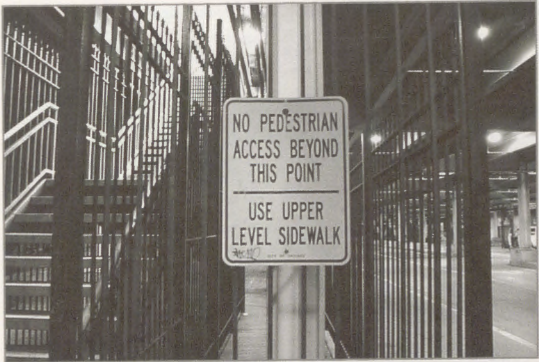
Figure 51. Fencing restricting pedestrian access on Lower Wacker Drive in response to the homeless encampments.
