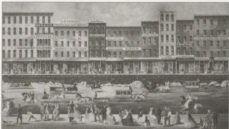
Figure 26. Street grade raising in progress in Chicago's Loop.
