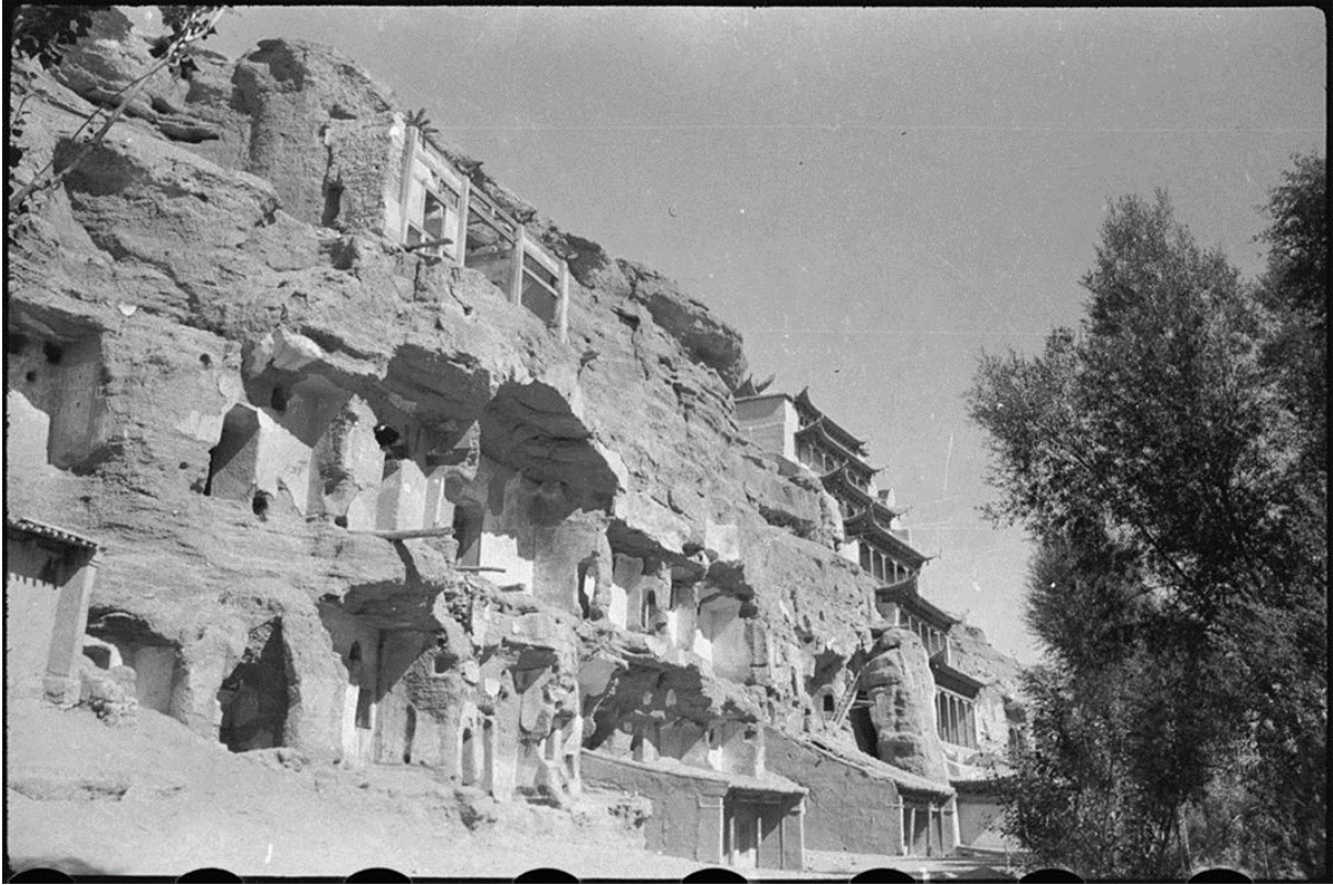
Figure 3-3. The area to the north of Cave 96 in 1943–44 showing the nine-story pavilion of Cave 96, the Qing-period ante-halls of Caves 98, 100, and 108 on the ground level, the late-Tang porch of Cave 196 on the third level, and the beams for the overhanging corridors that connect the exposed antechambers of the second level. Photo by James Lo in 1943–44. James and Lucy Lo Photograph Archive.
