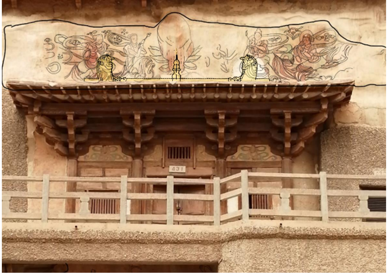
Figure 4-37. The timber-structured façade and open-air mural of Mogao Cave 431 overlapped with trace-copy line drawings and reconstructed ridge ornaments. Photo and drawing by author.
