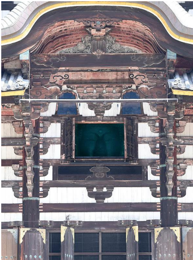
Figure 3-21. The high window above the entrance of the main Buddha hall of Todai-ji, Nara, Japan. Initial construction completed in 751, current structure rebuilt in 1709. Photo after Kato, “Nara’s Todaiji Temple Closed.”
