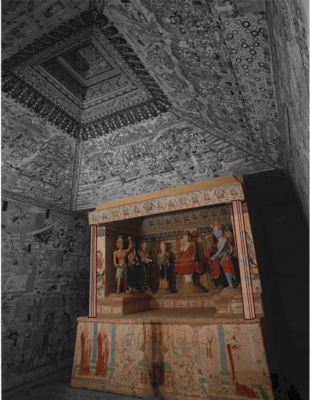
Figure 2-27. The central pillar in the shape of a canopy, Mogao Cave 9, late-Tang period, showing author's theoretical reconstruction of the canopy lintel and posts in brown lines and translucent colors. After Sun and Sun, Shiku jianzhu juan , 117, fig. 80. Photo processed by author.
