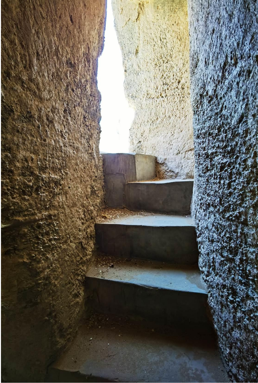
Figure 5-33. A tunnel to north of Cave 234 for vertical circulation at the Mogao caves, with modern renovation of the stairs. Photo by author, 2021.
