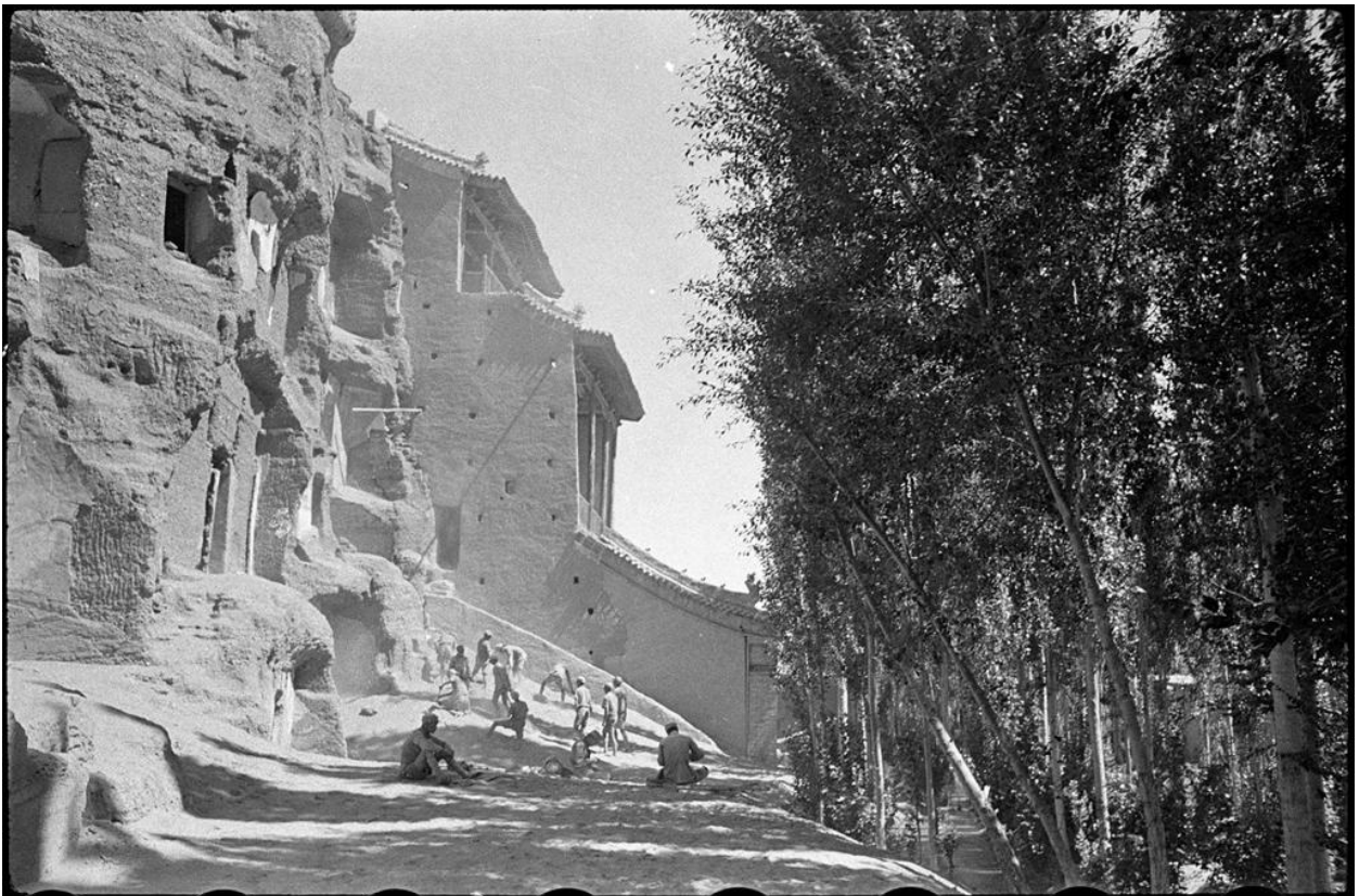
Figure 0-2. The three-story pavilion, seen from the south side. Photo by James Lo, 1943–44. James and Lucy Lo Photograph Archive.
