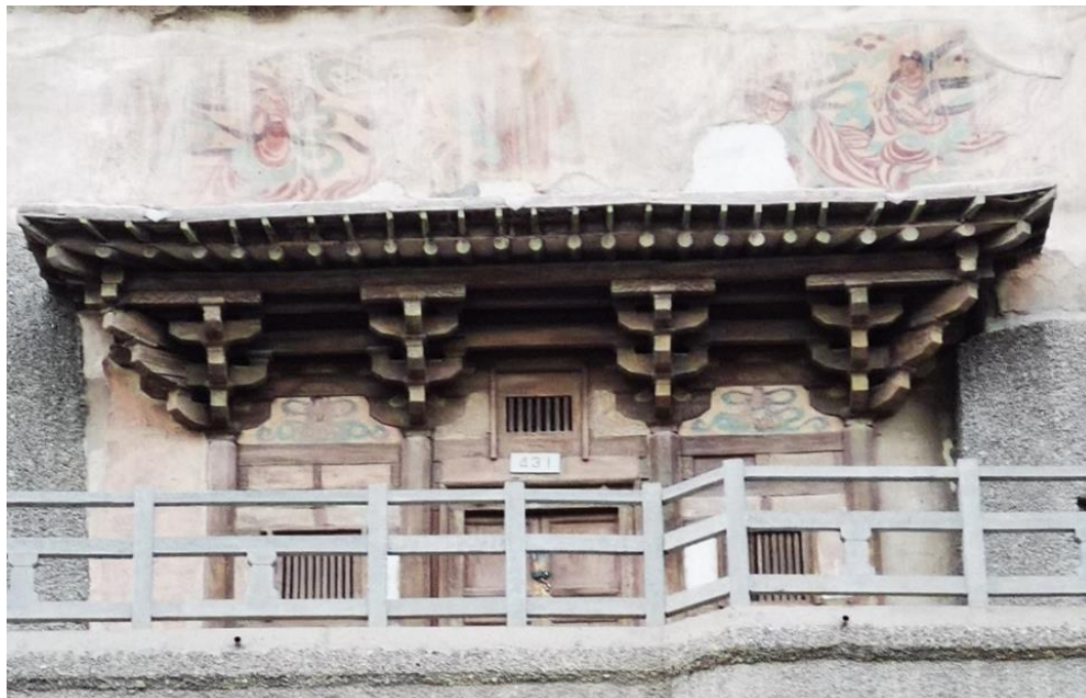
Figure 3-2. The timber-structured façade and exterior mural of Mogao Cave 431 showing three-step bracket-sets, a three-bay façade, and an overhanging roof. Dated by inscription to 980 CE. 486 cm (w) × 142 cm (d) × 320 cm (h). Wood, mud brick, polychromic pigments. Photo by author, January 20, 2022.
