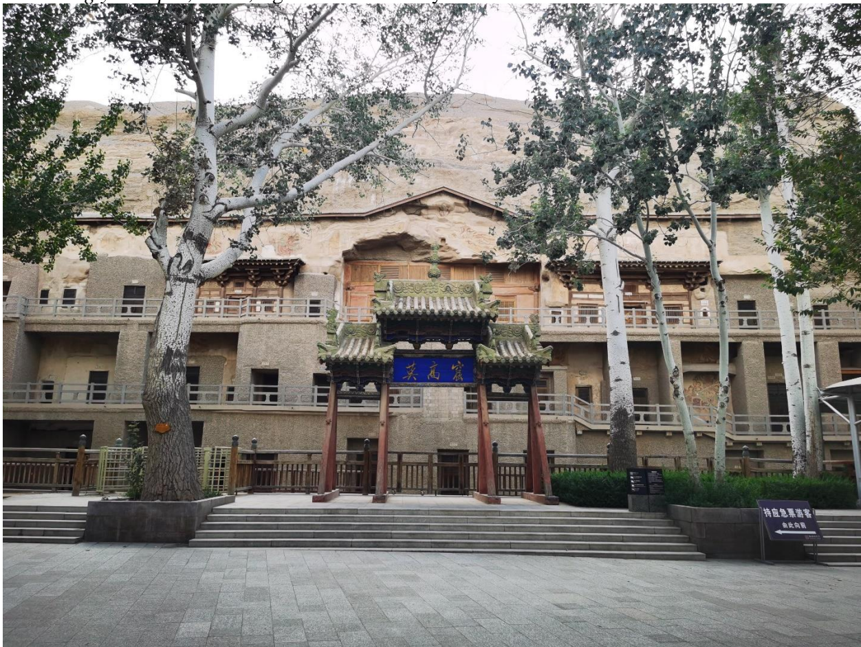
Figure 4-34. A recent photo of the area around Cave 428. The decorative gateway was constructed in the Qing dynasty, the roof that shelters the open-air murals added in the 1950s, and the concrete passageways in the 1960s. Photo by author, March 2022.
