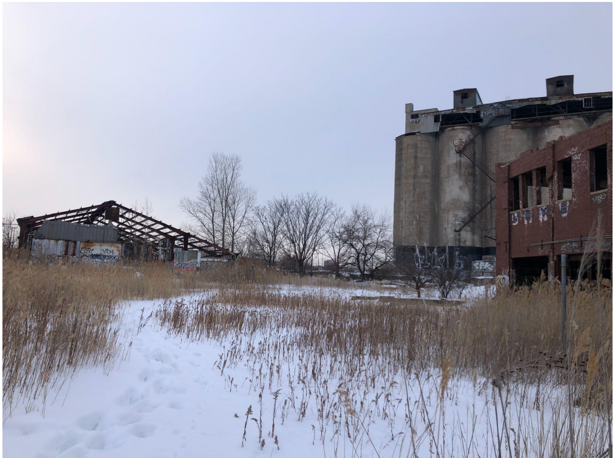
Figure 6: Damen Silos, February 2021 68
