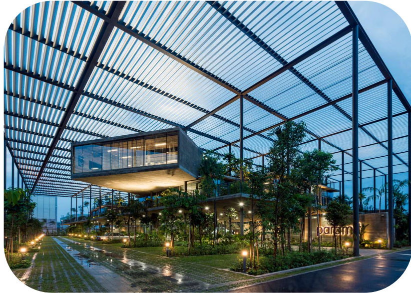
Figure 10: "Factory in the Forest," Malaysia. A prime example of biophilic architecture. Image credit: Ho (2017).
