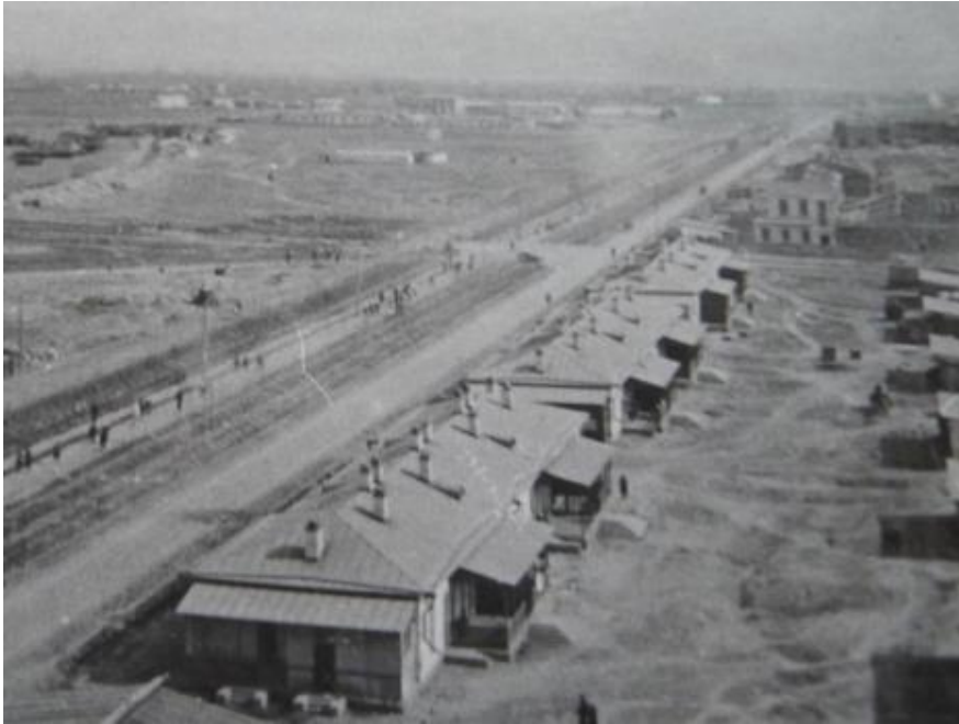
Figure 24: Aerial view of central Stalinobod in the 1930s.
