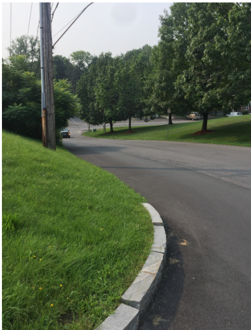
Figure 2. Photograph of an inaccessible “approach to the building” (taken by Carolyn)
