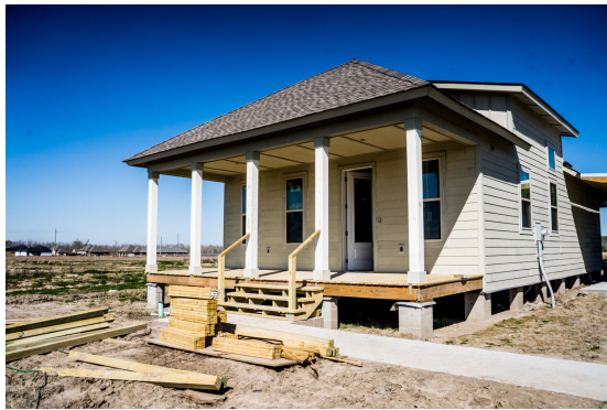
Figure 6: Partially constructed houses on the New Isle fared well after Hurricane Ida Source: Setyawan 2021
