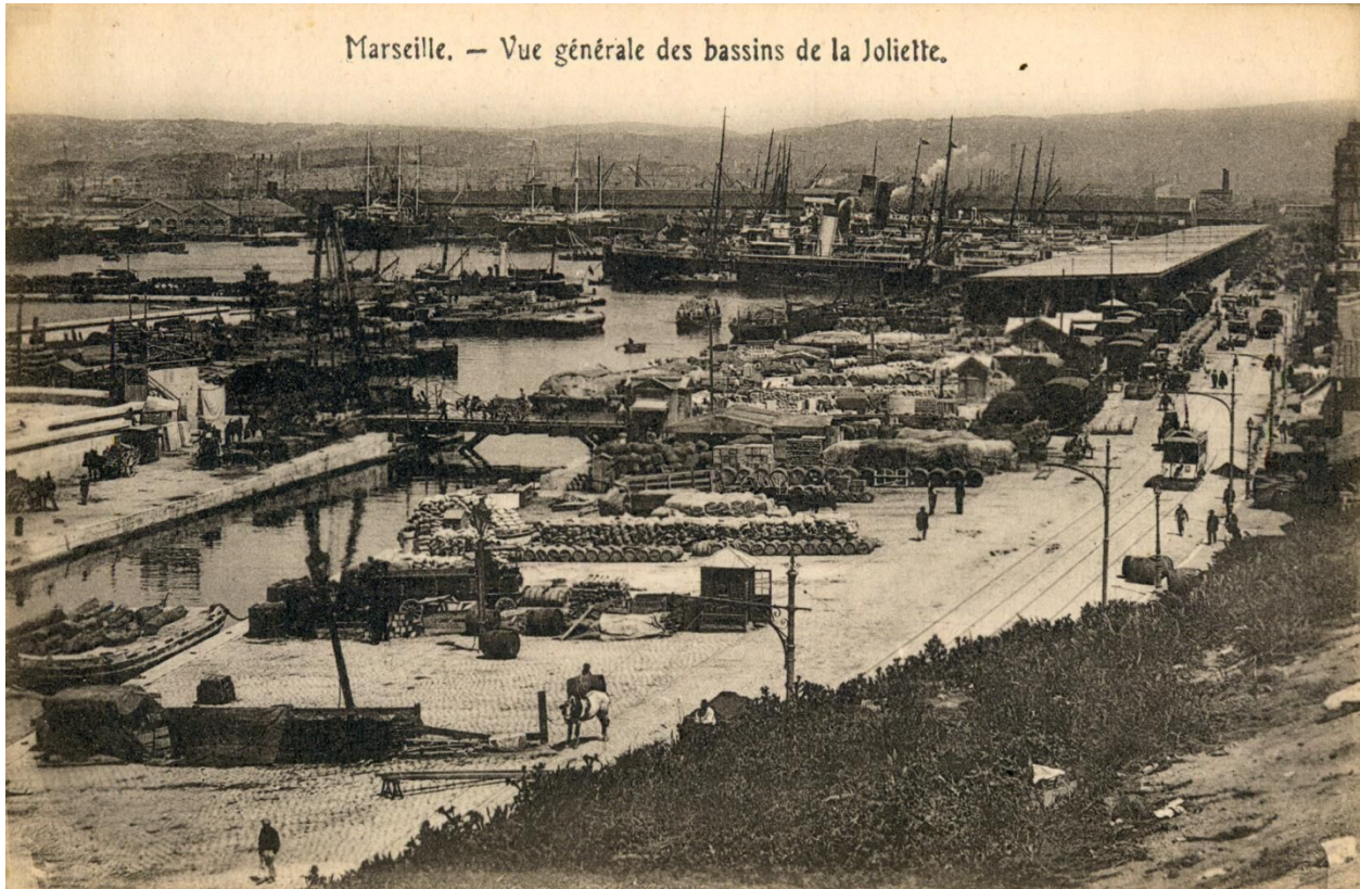
Figure 16: The newly-constructed bassin de la Joliette , built on reclaimed land created with soap factory waste. 283
