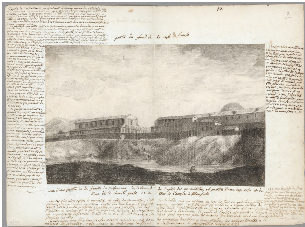
Figure 7: Soap factory in l’anse de l’ourse, late-eighteenth century. This illustration shows the artificial slopes, described in Péclet’s account, that were created by the disposal of soap factory waste in the cove. 155
