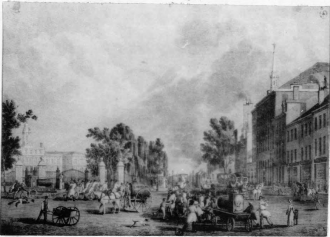
Fig. 35--J. W. Hill, "City Hall and Park Row."
