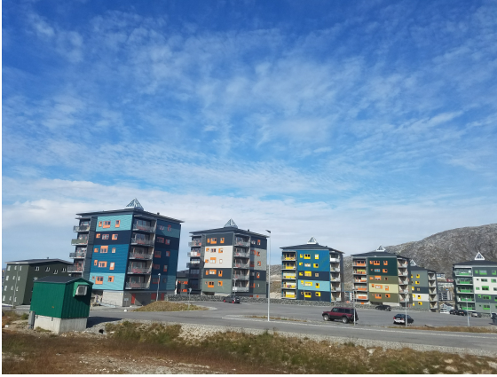
Figure 1.5: Newer apartments in Nuuk
