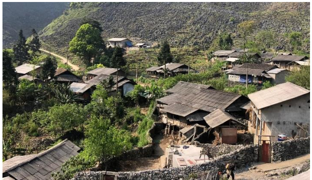
5.10. A village where all stilt houses have corrugated iron roofs, and some concrete houses
