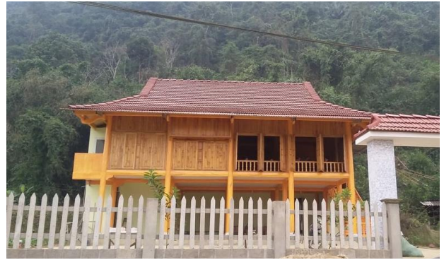
5.6. Finished concrete stilt house
