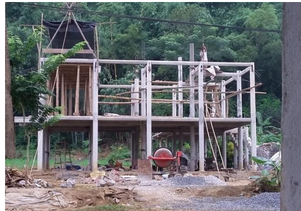
5.2. Frame of a concrete stilt house
