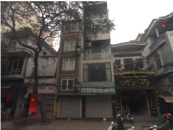
3.1. The façade of a tube-house row in Hải Phòng
