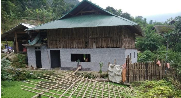
5.5. Traditional stilt-house with corrugated iron roof and partially concrete wall
