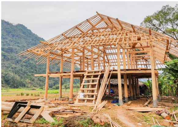
5.1. Frame of a wooden stilt house
