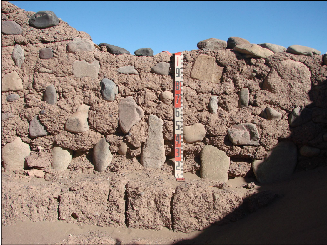
Figure 3. 6. Ramaditas, Compound I, Structure 4 (N wall), shows a long building sequence: an excavated interior surface, stones slabs that provide the foundations for the aerial portion of the wall, which combines large stones with mortar.
