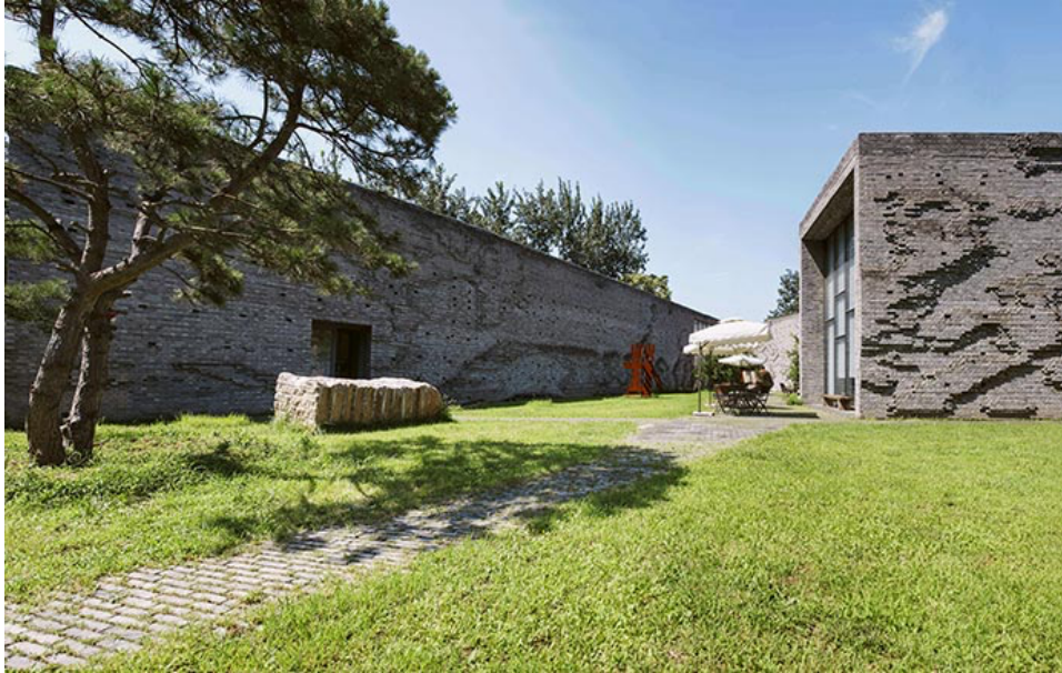
Fig. 3.47: Three Shadows Photography Arts Centre designed by Ai Weiwei, 2005, Beijing. Entrance door shown to the left.
