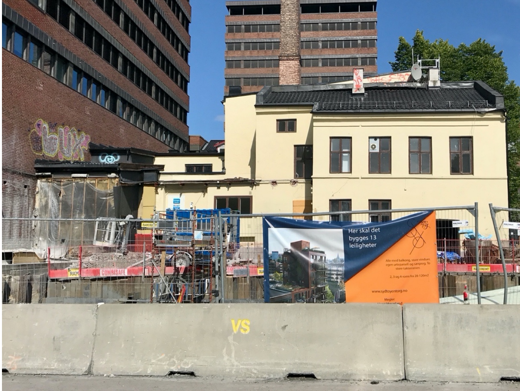
Figure 5.1: South Tøyen Square construction site as seen from Hagegata, with the old yellow building and the 1970s towers in the background. Photo by author.
