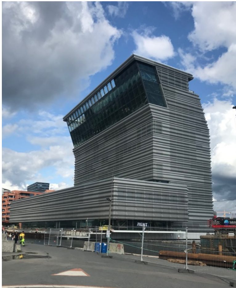
Figure 4.7: Lambda building under construction. Photo by author.
