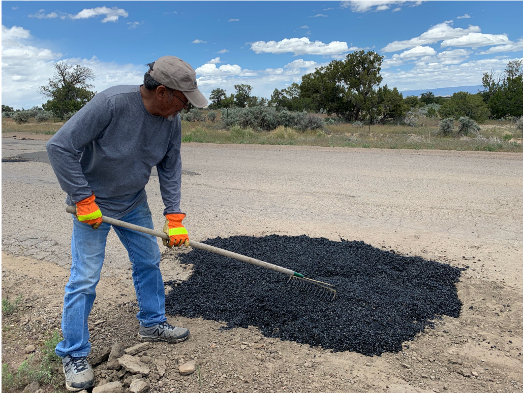
Figure 13 - George patching a medium-sized hole: the raking step.
