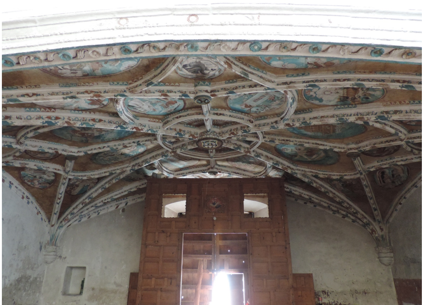
Figure 3.24. Don Juan Gerson. Apocalypse Cycle . Pigment on amatl . Soffit, church of Nuestra Señora de la Asunción, Tecamachalco, May 1562. Photo by author.
