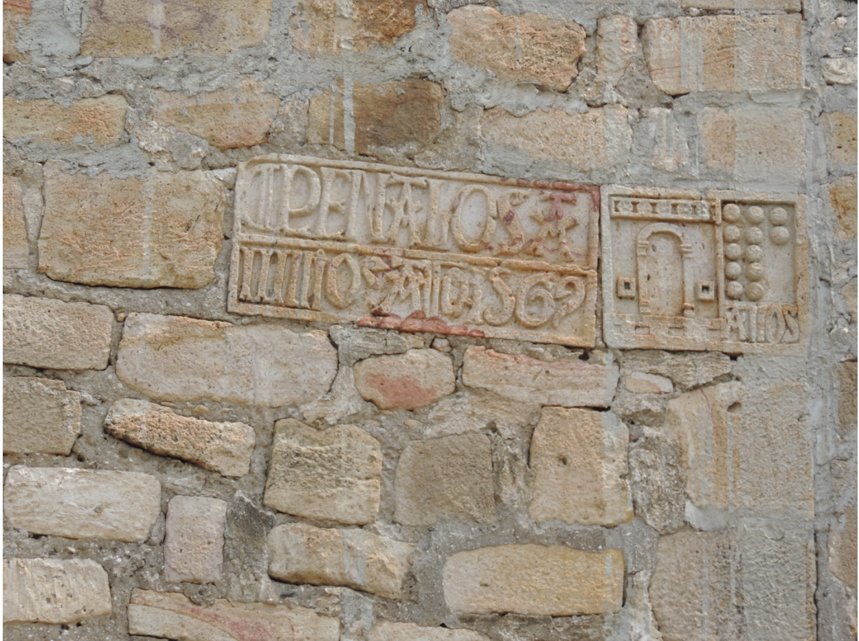
Figure 1.30. “D. PENALOSA / JULIOS AÑO 1569. East cloister façade. San Martín de Tours, Huaquechula, ca. 1569. Photo by author.
