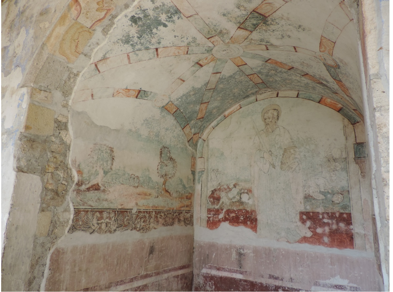
Figure 4.2. West wall. Oratory 4. Upper cloister. San Martín de Tours, Huaquechula, ca. 1569. Photo by author.
