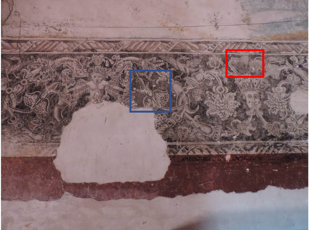
Figure 3.21. Detail: Sotocoro , north wall. A philodendron is in the blue box and morning glory is in the red box. Church of San Martín de Tours, Huaquechula. Photo by author.
