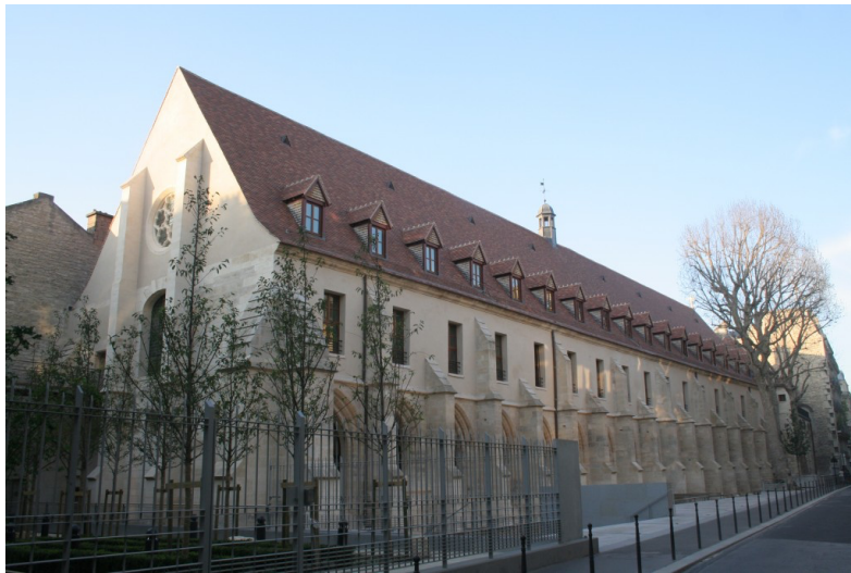
Fig. 4.7 Interior and Exterior of the Refectory, Collège des Bernardins, begun 1248, Paris
