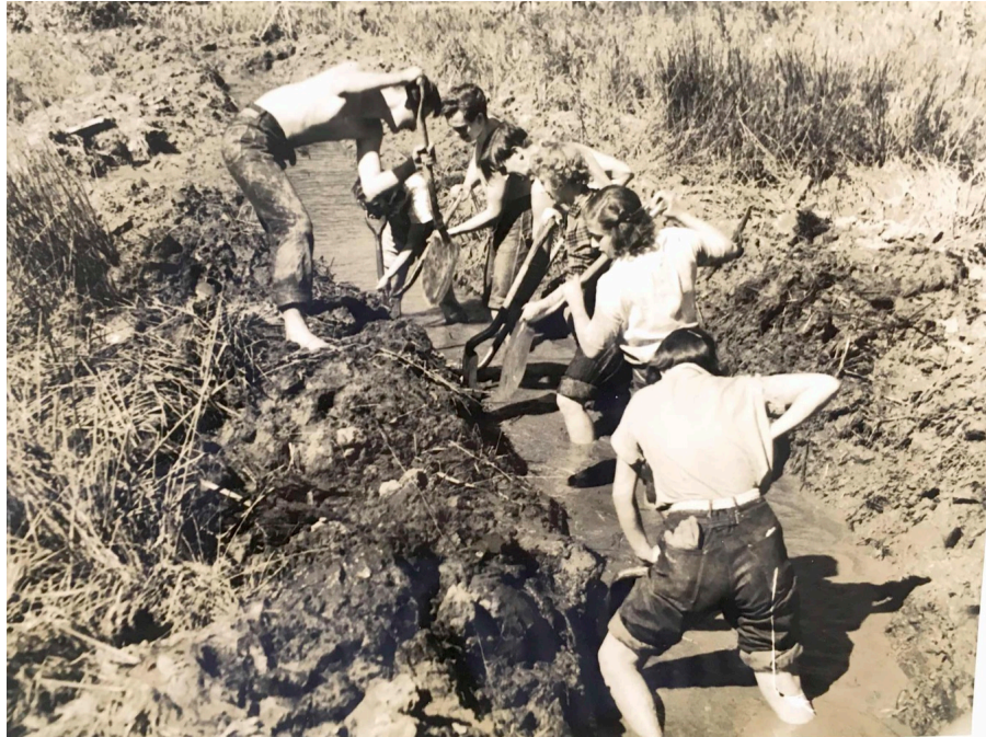
[fig. 3.19] The spirit of work: Student workers digging a drainage ditch, 1940
