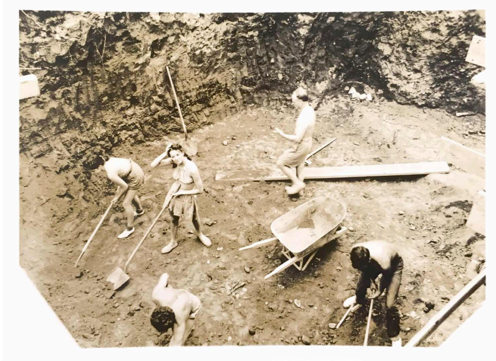
[fig. 3.14] Theodore Dreier leading construction on the Studies Building foundation, 1940
