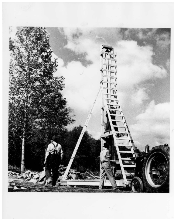
[fig. 3.17] Dreier and Charles Godfrey’s tractor-powered pile-driver, 1940
