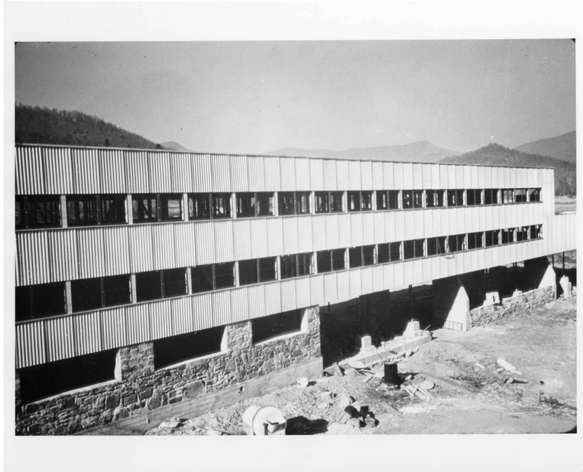
[fig. 3.15] Studies Building under construction, 1941
