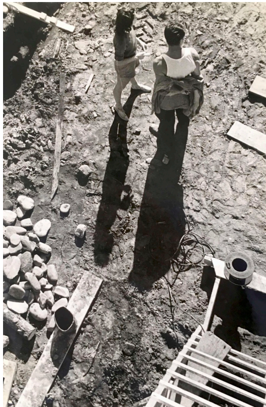
[fig. 3.20] The spirit of work: Student workers take a break while
