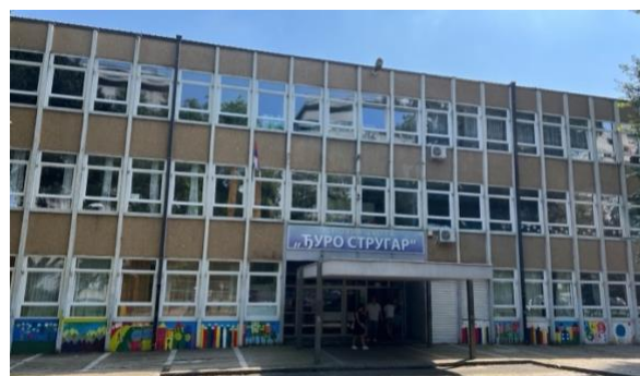
Figure 4. Elementary school in Blok 37.
