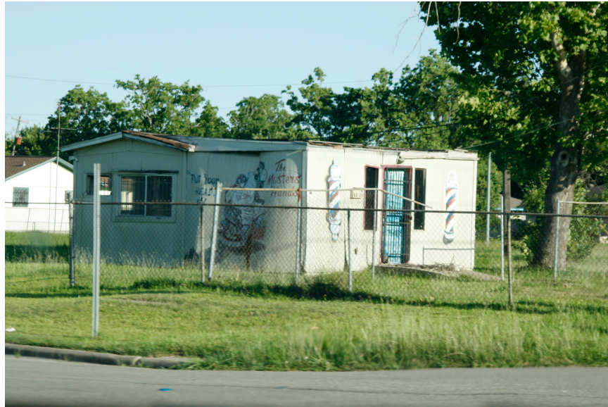
Figure 9. A one-room barbershop surrounded by a chain-link fence. Photo by author, 2014.
