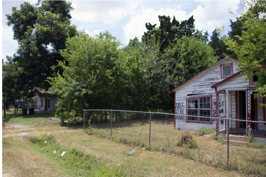
Figure 1. Original wooden-framed house with an open ditch in front. Photo by the author, 2014.
