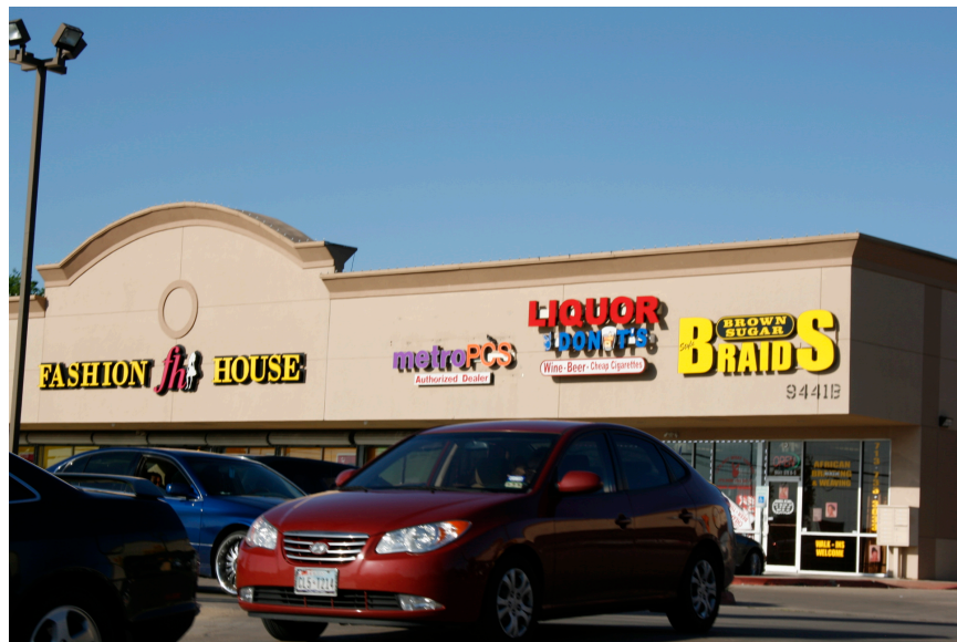
Figure 11. Commercial shops in Cullen Plaza, the primary commercial strip in Sunnyside. Photo by Laurence Rice, 2014.
