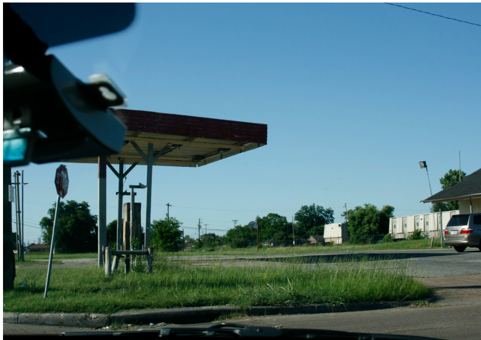
Figure 17. Abandoned gas station near Scott Plaza Apartments. Photo by the author, 2014.
