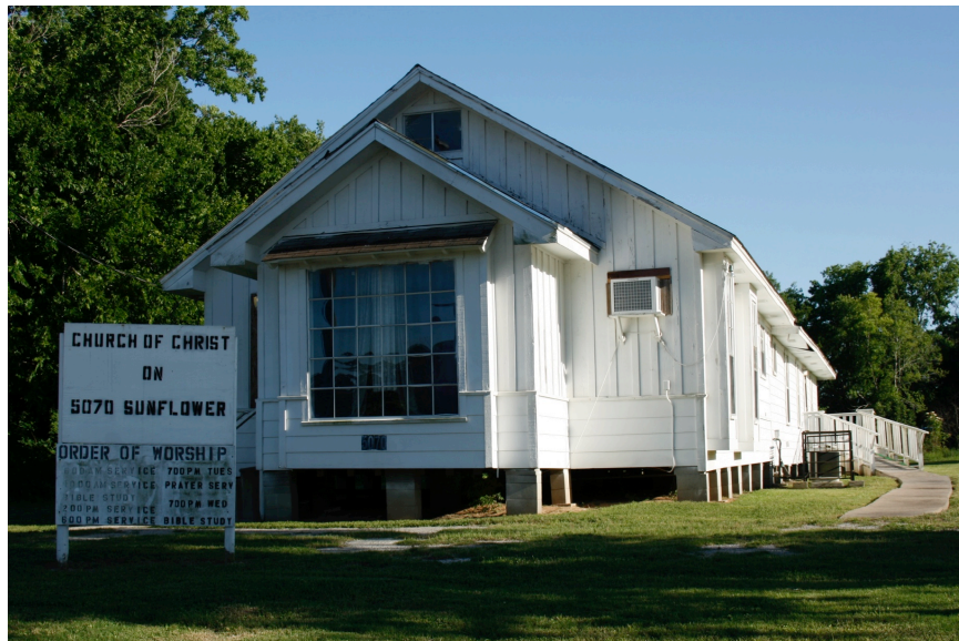
Figure 3. Church of Christ on Sunflower Street, set up on cinder blocks. Photo by the author, 2014.
