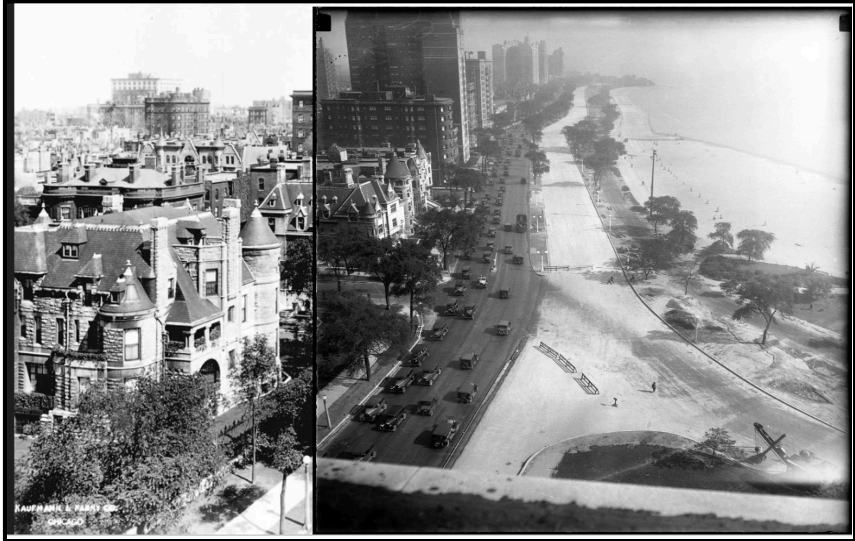
Figure 4: Lake Shore Drive, Looking North from the Drake Hotel . DLSD during expansion (1927) with referenced photo overlay, from the Chicago Tribune. 43
