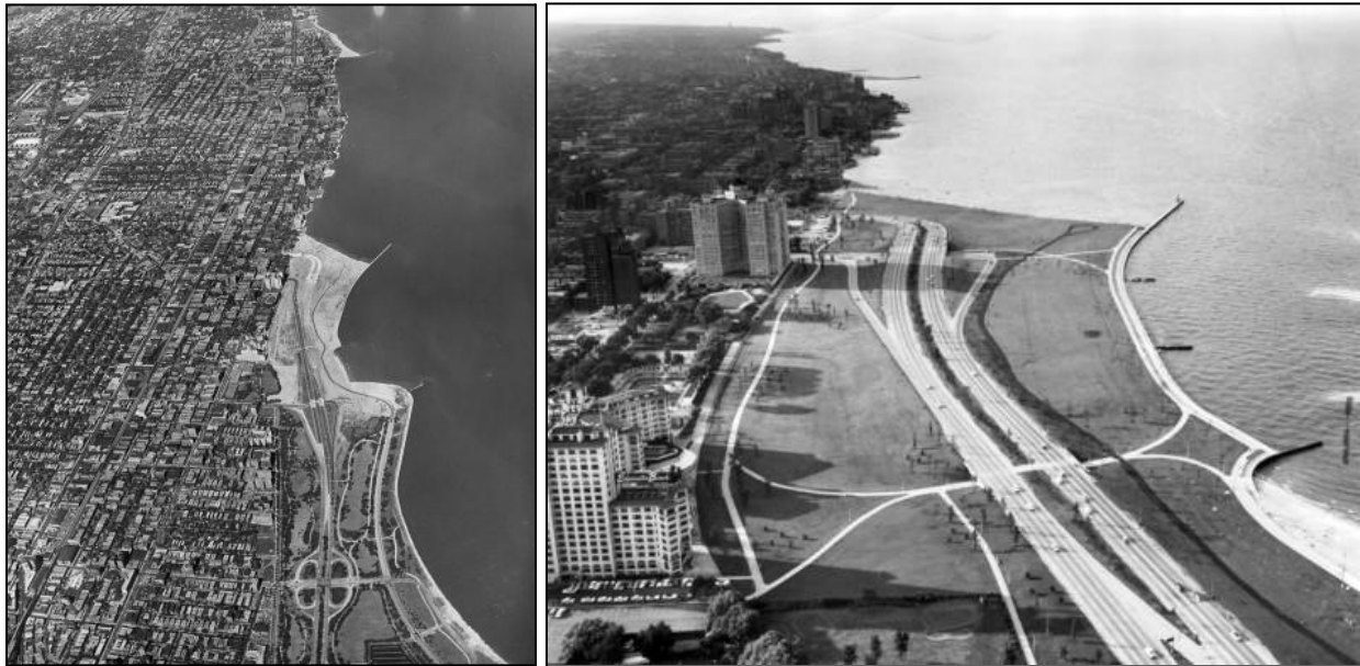
Figure 5: DLSD's Hollywood Avenue Extension during (early 1950s, left, from the Chicago Historical Society) and after (1958, right, from the Chicago Tribune) construction. 48
