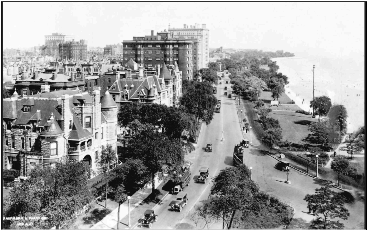
Figure 3: Lake Shore Drive South of Lincoln Park . DLSD in 1920, before expansion, from the Chicago Tribune 42
