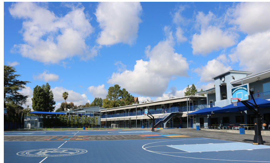
Photographs: [Top] Chamlian’s renovated blacktop yard, which now boasts astro-turf fields, and repainted athletic courts. [Bottom] Chamlian’s several classroom buildings in view, with repainted basketball courts in the foreground.
