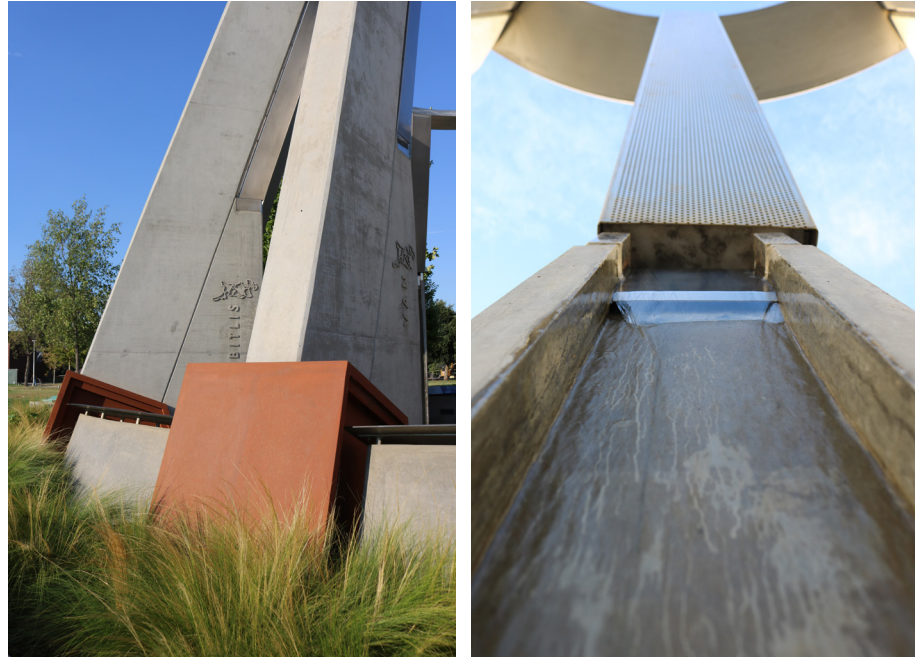
Photographs: [Left] Columns of the Armenian Genocide Monument, featuring tufa stone bases and plants native to Armenia [Right] Inside the columns, featuring flowing water canals
