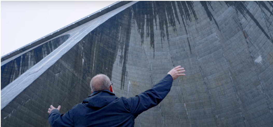
Image 20: Nærbø stands beneath one of Manic-5's thirteen arches. from Scalability of hydropower , 0:30.
