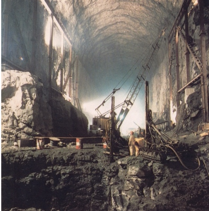
Image 28: Excavation of the Churchill Falls powerhouse. from Brinco , photo insert 1, page 10.
