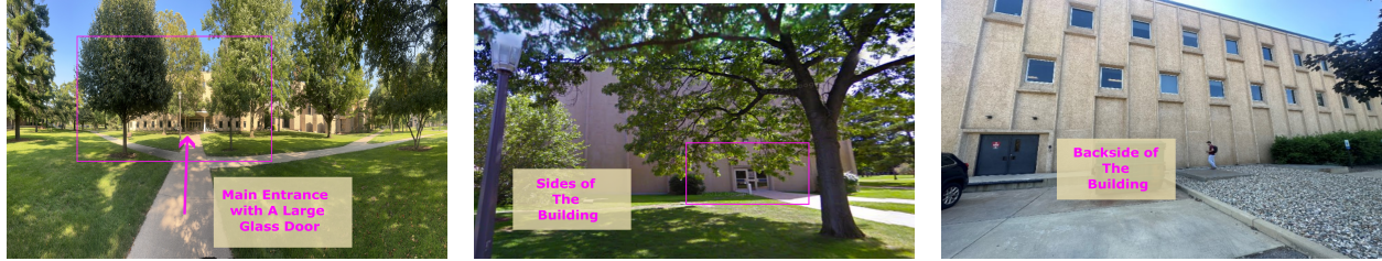
(a) Frontside of the measurement building: With a large glass door. (b) Sides of the measurement building: With a glass door, no windows. (c) Backside of the measurement building: No windows on the first floor.
