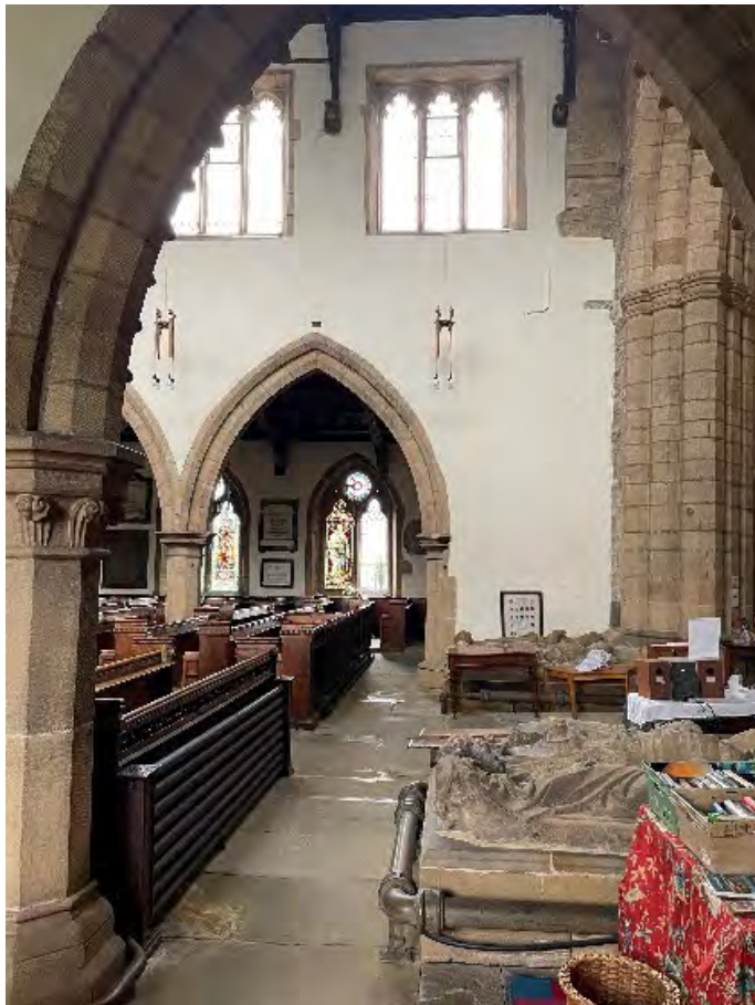
FIG 2.37 View toward south aisle of St Gregory's Church
