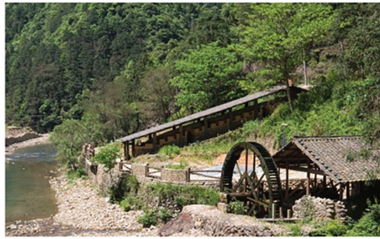
A Dragon Kiln Structure in Longquan Kiln, Zhejiang
