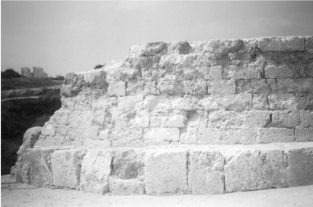
Figure 7. “Craters” from direct catapult hits on the face of the southern gate tower (photograph: Yotam Tepper).
