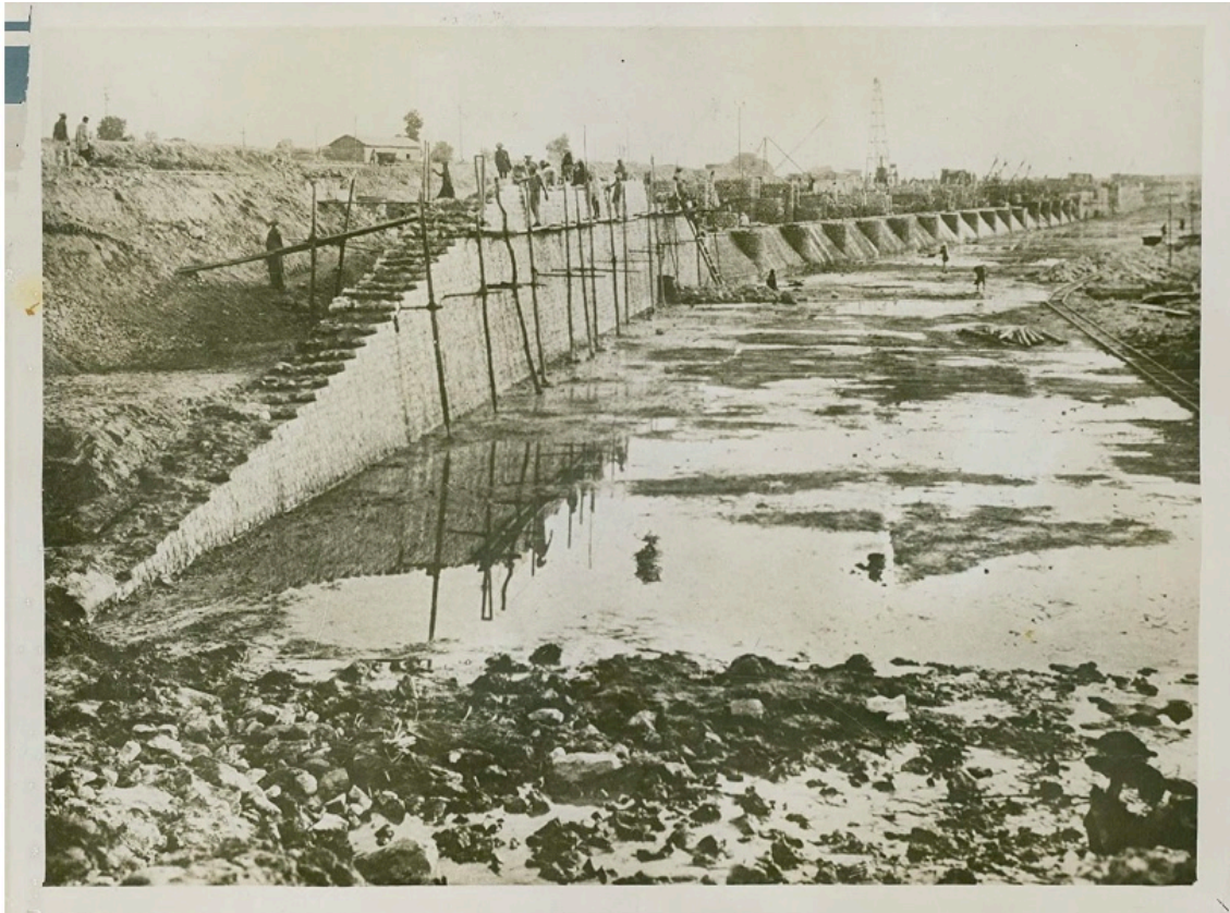
Figure 3. Working on the Sukkur Barrage
