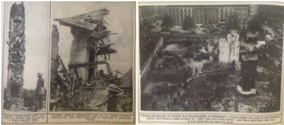
(Figure 2.4 (left): “German observation post constructed within the hollow of a shell-broken tree.” Figure 2.5 (center): “Concrete German observation post at la Bassée cleverly camouflaged with shattered roof to simulate a worthless house.” Figure 2.6 (right): “Trafalgar Square, in London, was transformed to represent a war-scarred village on the Western Front, and people were invited to ‘feed the guns with bonds’ and thus help end the war.” Reproduced from The War of the Nations .)
