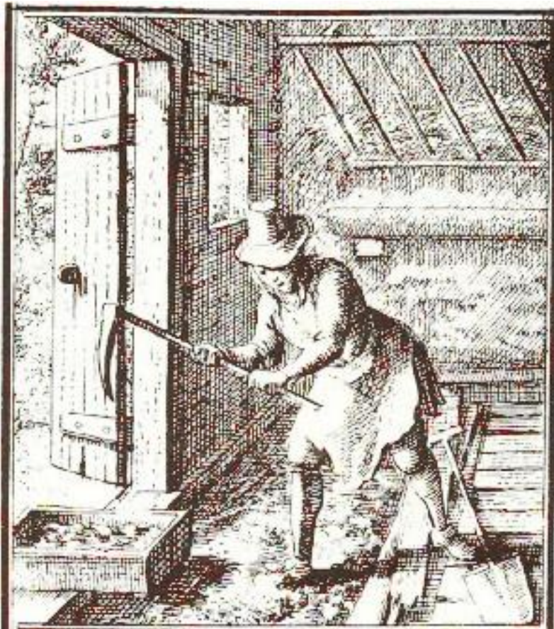
Figure 1.1, Saltpeterman digging under stable, mid-16th century (Source: Wikimedia Commons).
