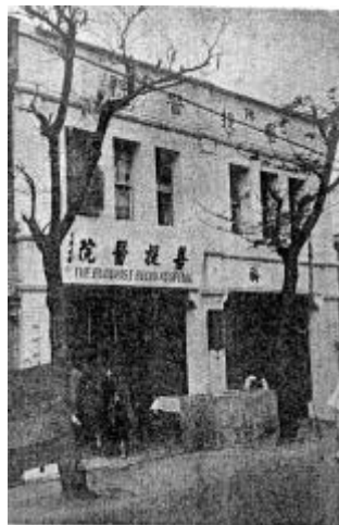
Figure 5.1: The First Puti Hospital Building in 1963
