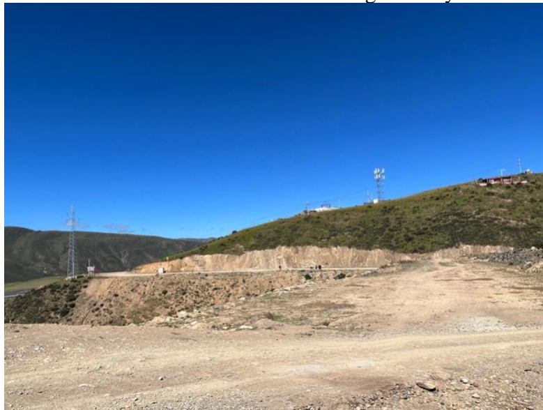
Photo 11 construction at Larung Gar Sky burial site
