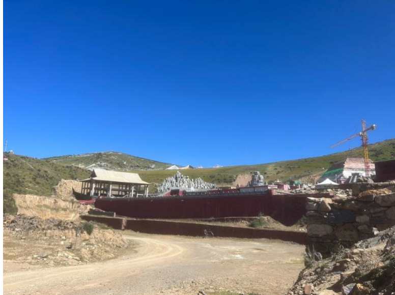
Photo 10 Construction at Larung Gar Sky Burial Site
