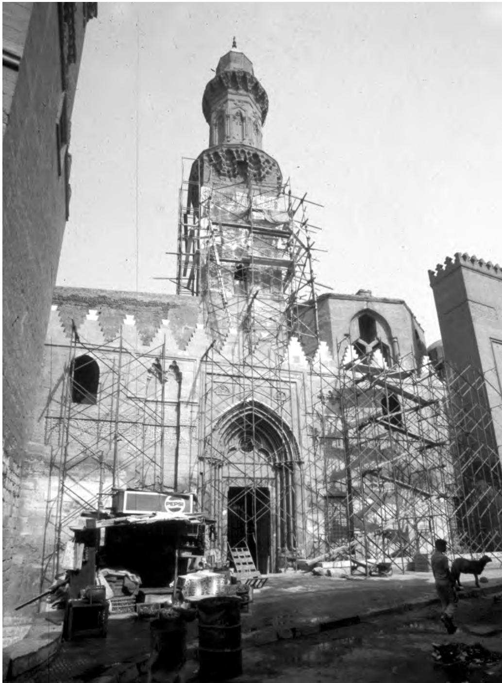
Fig. 10. Madrasah of al-Nāṣir Muḥammad, street elevation during restoration, 1986 (Speiser)
