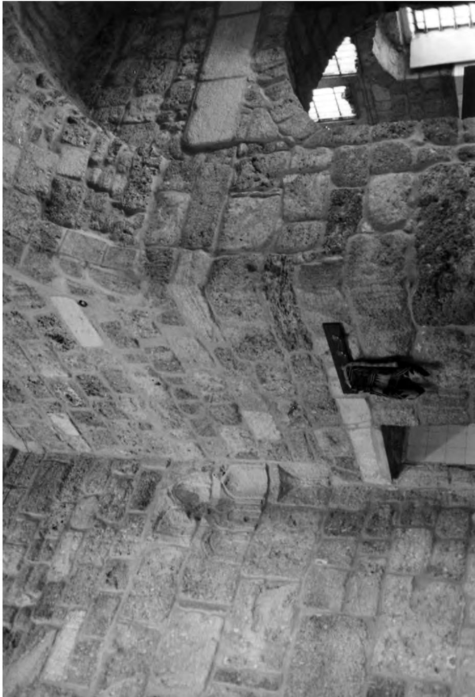
Fig. 8. Tripoli, 'Aṭṭār Mosque. View of the interior with the entrance to the ablution room from the prayer hall (B2): inserted muqarnas on the supporting pillar of the cupola. Photograph: Miriam Kühn, 2004.
